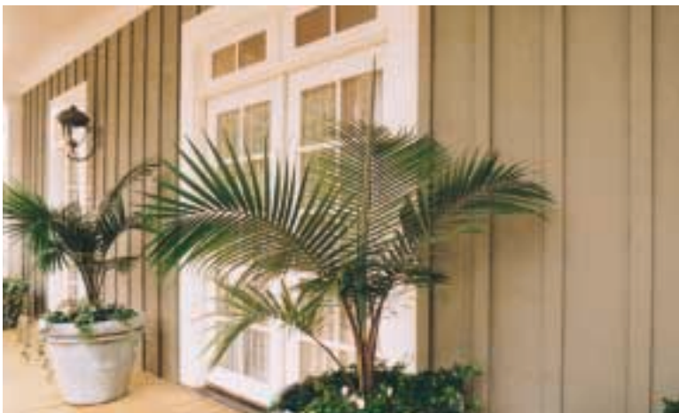
Painted 12 in. boards with 3 in. battens.
