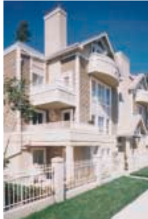
Opaque stained 6 in. bevel siding and cedar trim boards with stucco accents.
