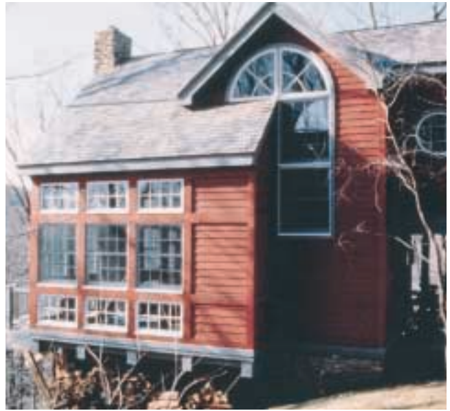
Opaque stain on 8 in. bevel siding with 6 and 8 in. trim boards.
