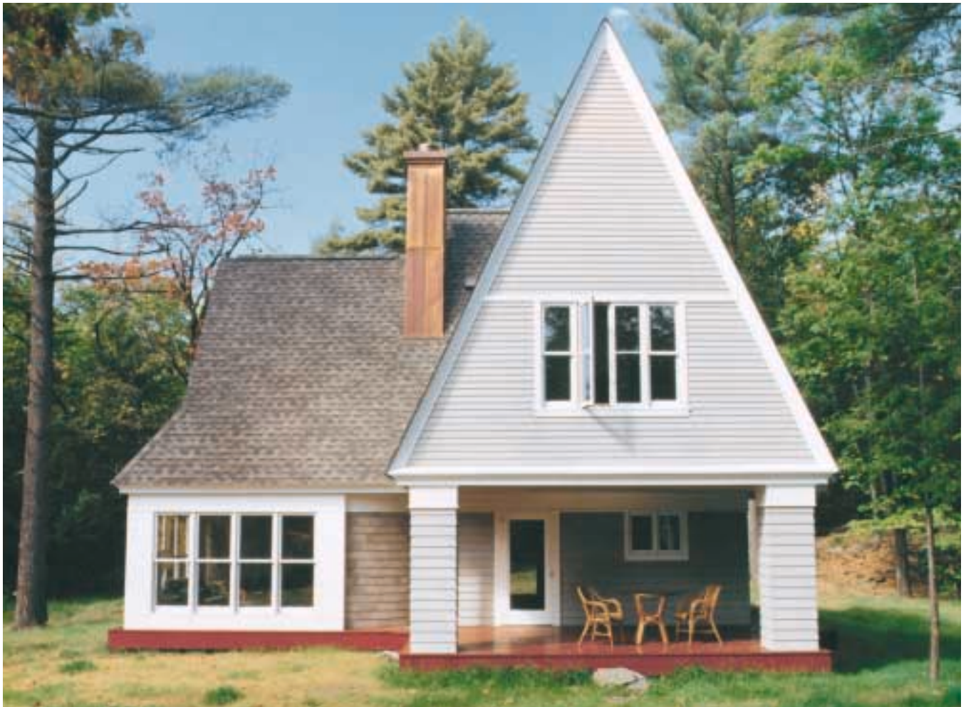
1x8 Western Red Cedar plain bevel on columns and 1x6 plain bevel on gable ends, finished with a grey stain. Cedar trim is painted white.
