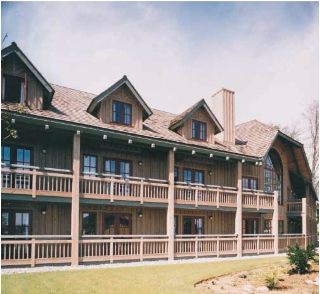
Board and batten siding on a waterfront fishing lodge. Light colored stain finish.
