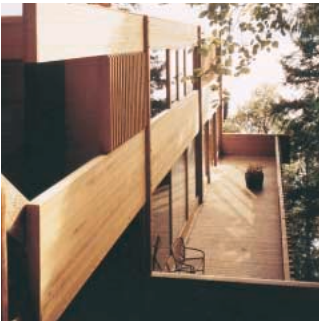
Horizontally applied clear 6 in. tongue and groove siding with natural semi-transparent stain.
