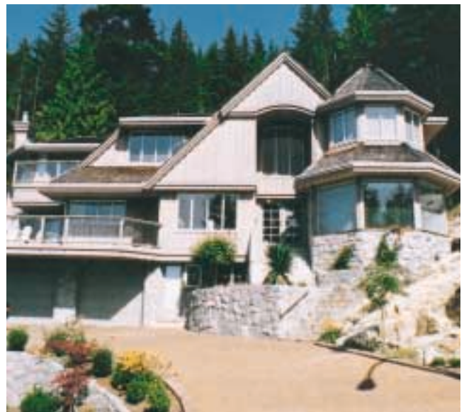
Ten-inch boards with 2 in. battens coated with driftwood grey stain.
