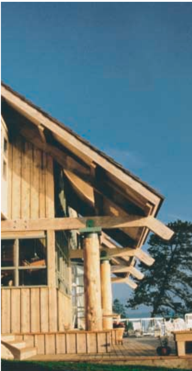
Ten-inch tight knotted cedar boards with 2 in. battens. Coated with clear water repellent preservative.
