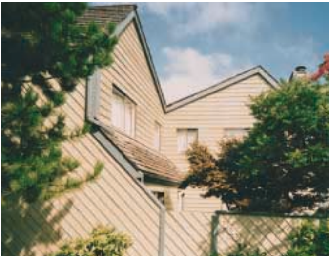
Eight-inch channel siding applied diagonally and horizontally and protected with opaque stain.
