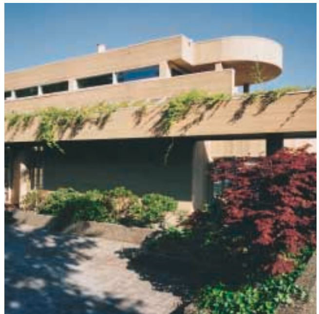
Horizontally applied clear 6 in. tongue and groove siding with natural semi-transparent stain.
