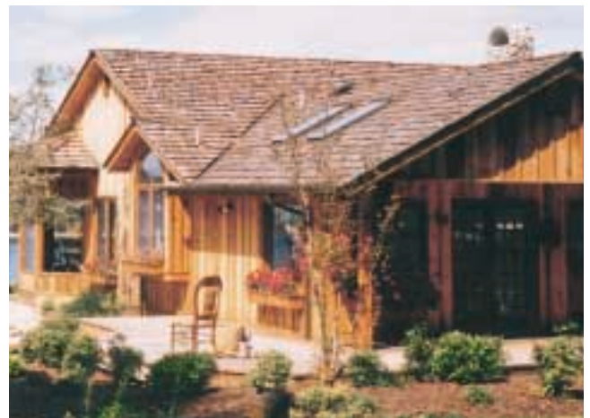
Ten-inch boards with 3 in. battens finished in a clear, water repellent preservative.
